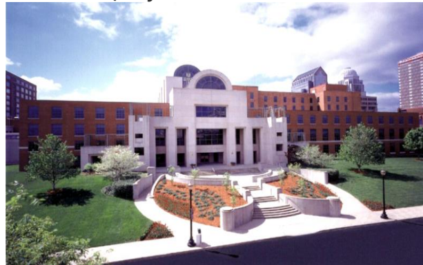
PCUSA Headquarters Building in Louisville, Kentucky. photo credit: PCUSA
